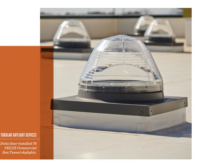
The reflectivity of tubular devices is crucial because some of the photons—or lightwave energy packets—are absorbed into the interior aluminum material of the tube with each angular bounce of light and converted into heat. However Sun Tunnels use an Almeco brand specular material that is nearly 100% reflective, so almost all the daylight collected on the roof is carried into the facility as light.
